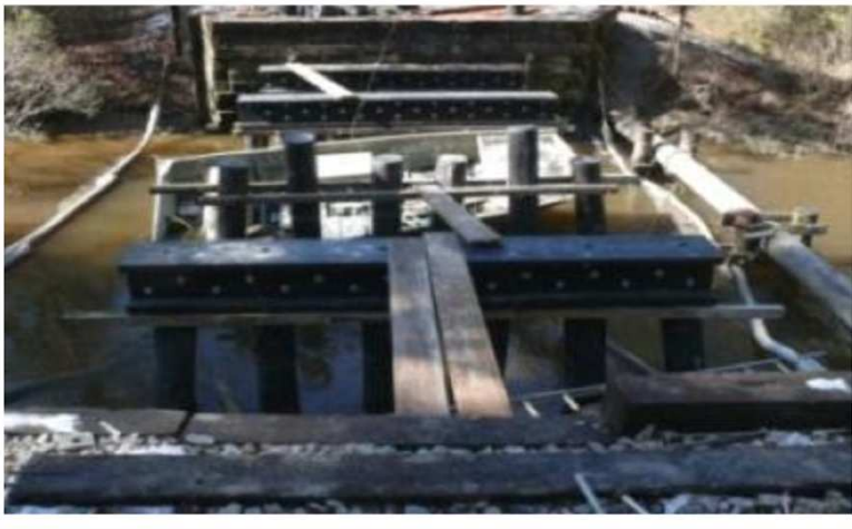
Pile Cap Installation
